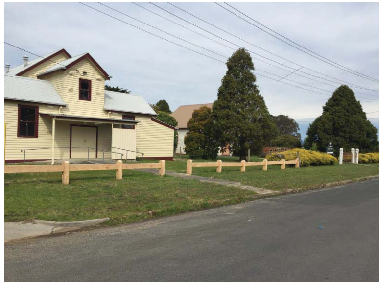
PHOTO 7 – Mechanics Institute Hall, St Johns Anglican Church and residential development in Railway Avenue
