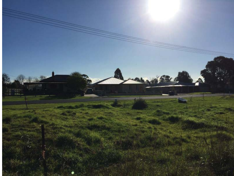
PHOTO 6 – Residential development on the west side of Main Street
