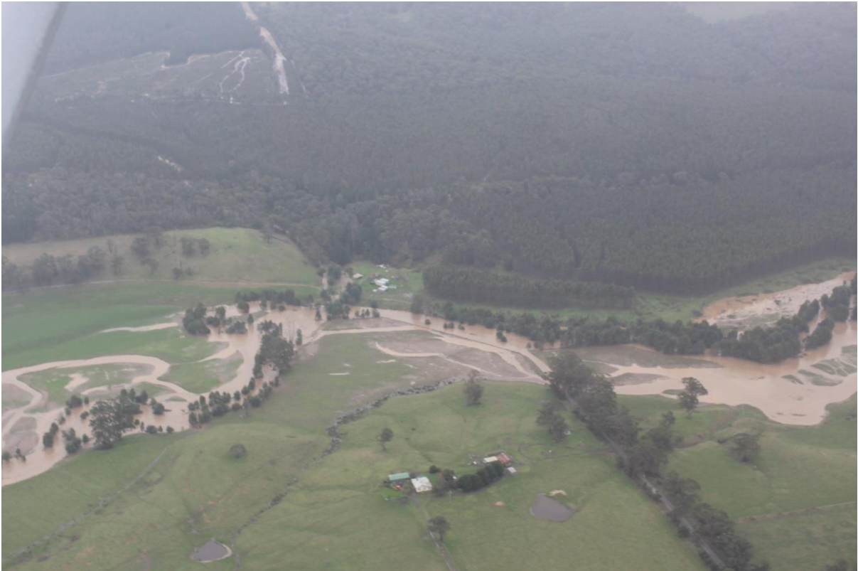
Figure 5 June 2012 Photography at Downies Lane Bridge
