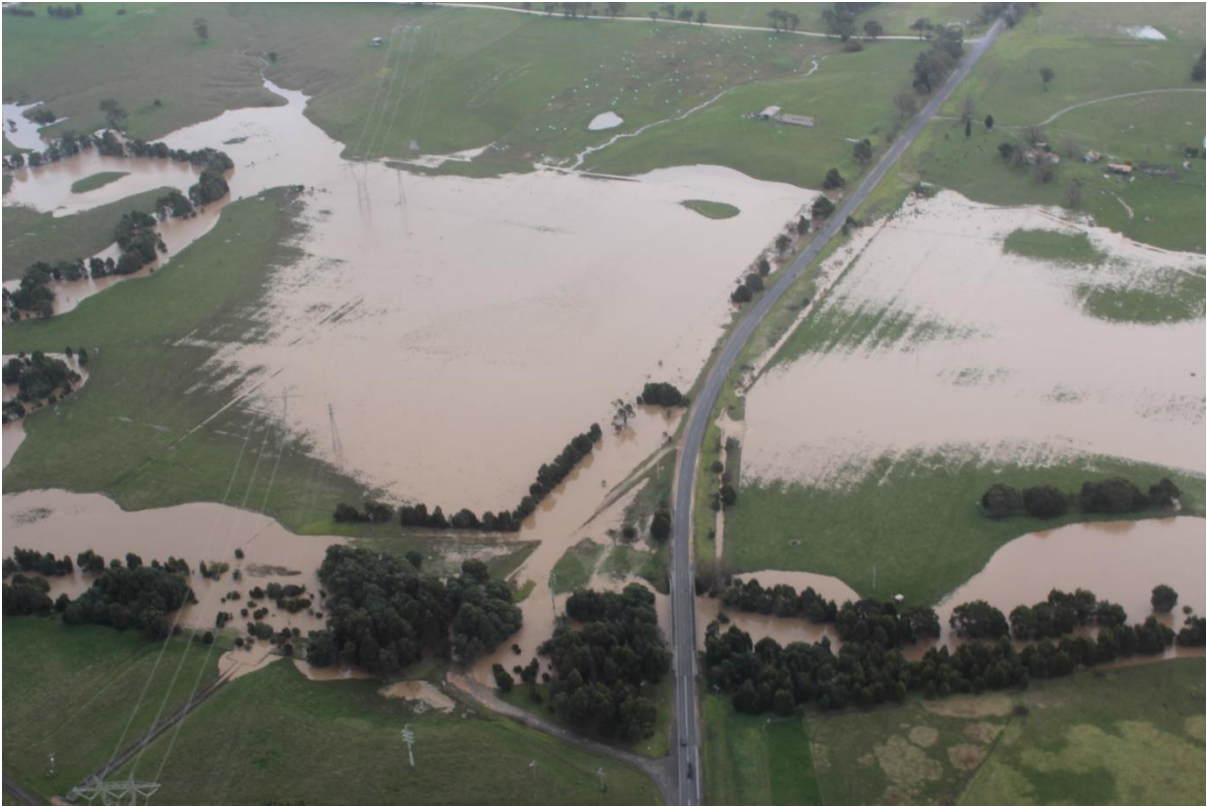
Figure 3 June 2012 Photography at Mattingley Hill Bridge
