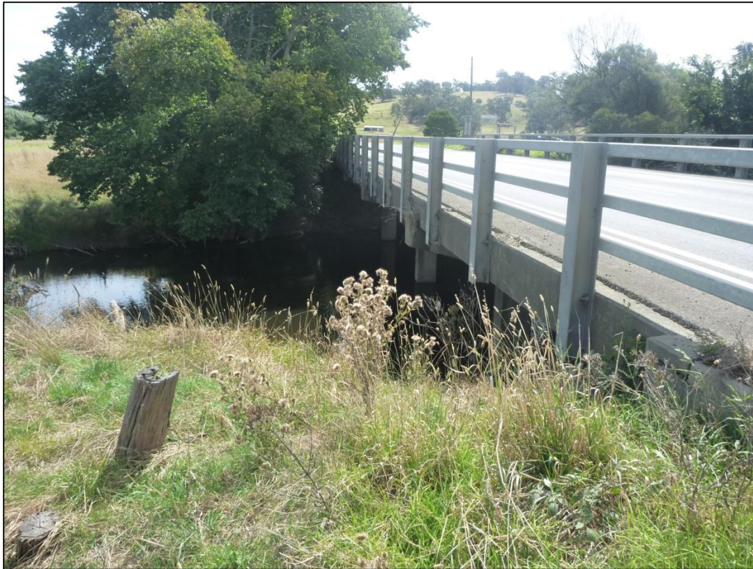
Figure 35 Brown Coal Mine Road south (downstream) side
