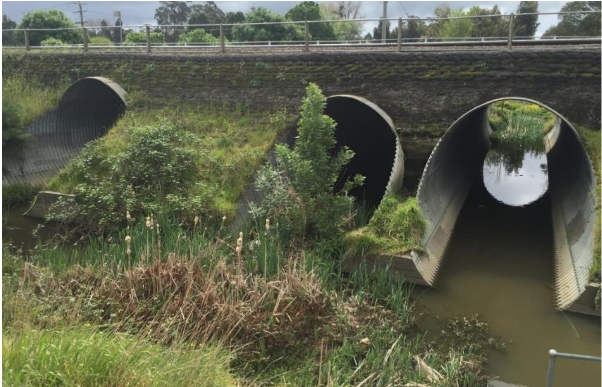
Figure 3-5 Traralgon Creek - Bairnsdale Railway Line Culverts (Looking North from Howitt St)
