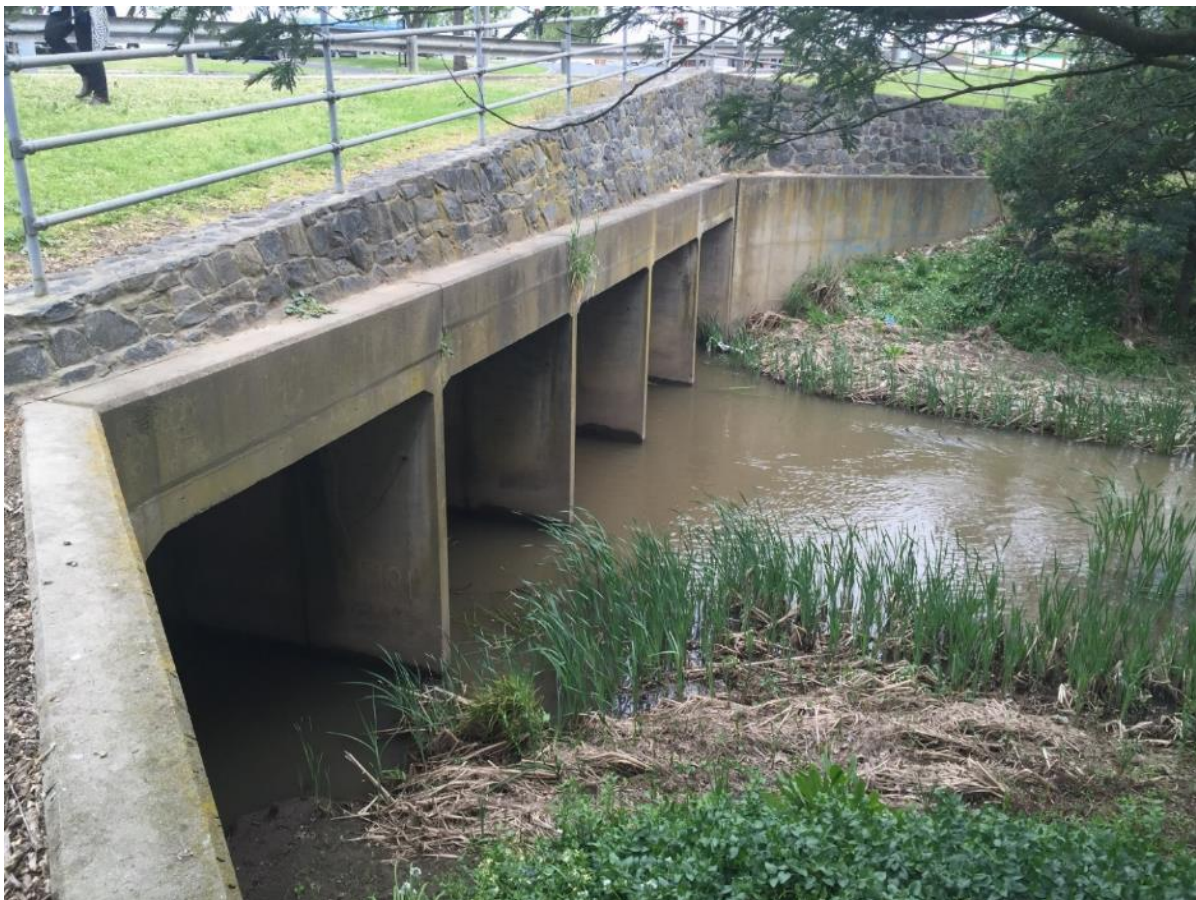
Figure 3-3 Traralgon Creek – Whitakers Road Culverts
