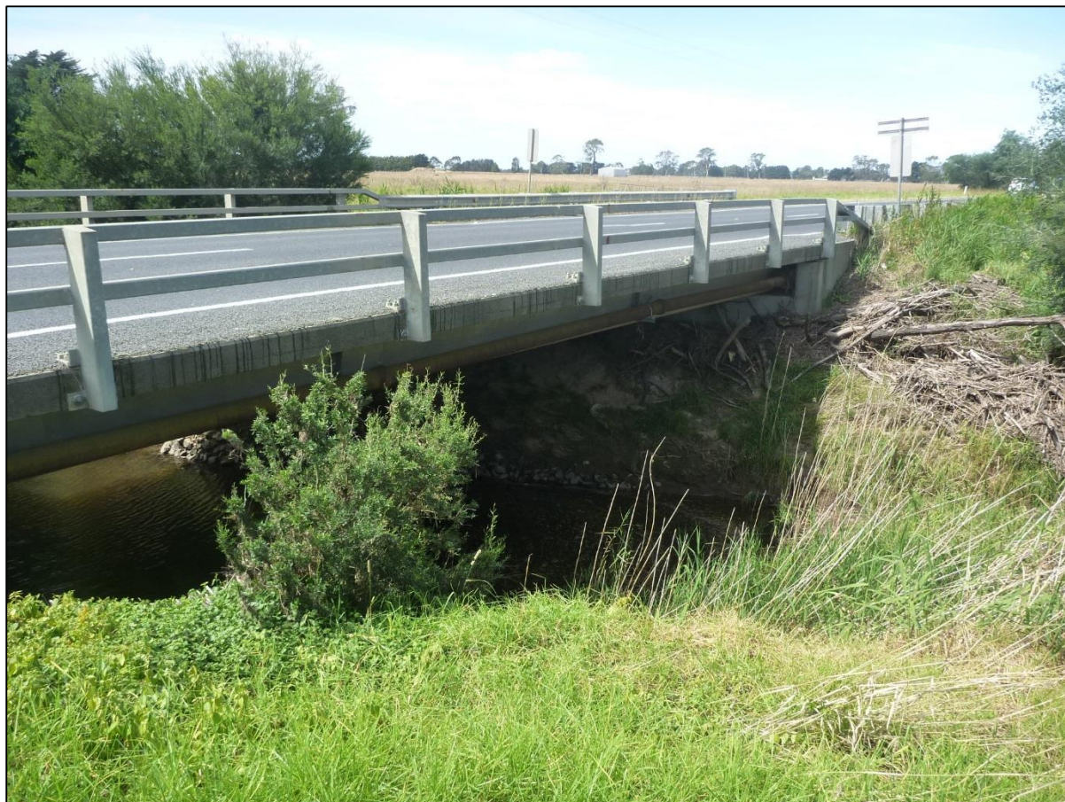
Figure 22 Bridge over Glengarry West Road
