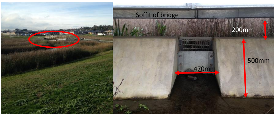
Figure 3-5 Eastern Wetland Outlet Arrangement (Source: WT site visit September 2015)
