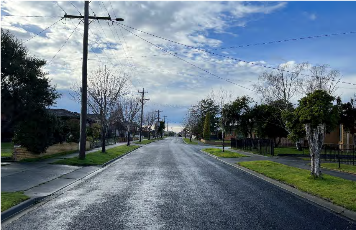
Photograph 1: Photograph of Ritchie Road. Demonstrates the 16m road reserve with footpaths and street plantings within.
