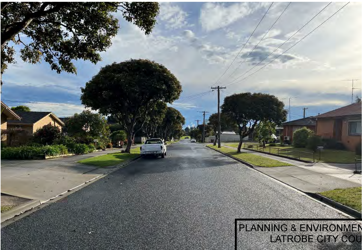
Photograph 4: Photograph of Manuka Crescent 16m wide road reserve.
