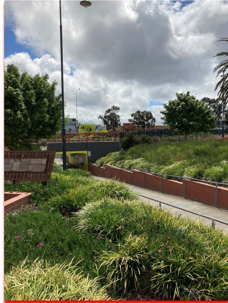
Pedestrian Underpass from Commercial Road
