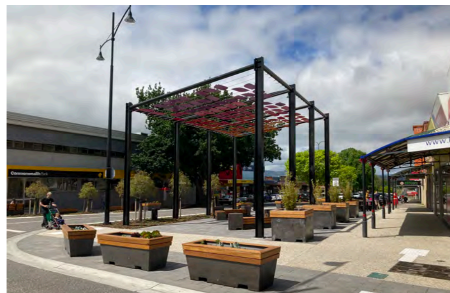
Recent streetscape works at corner of Tarwin Street and Commercial Road
