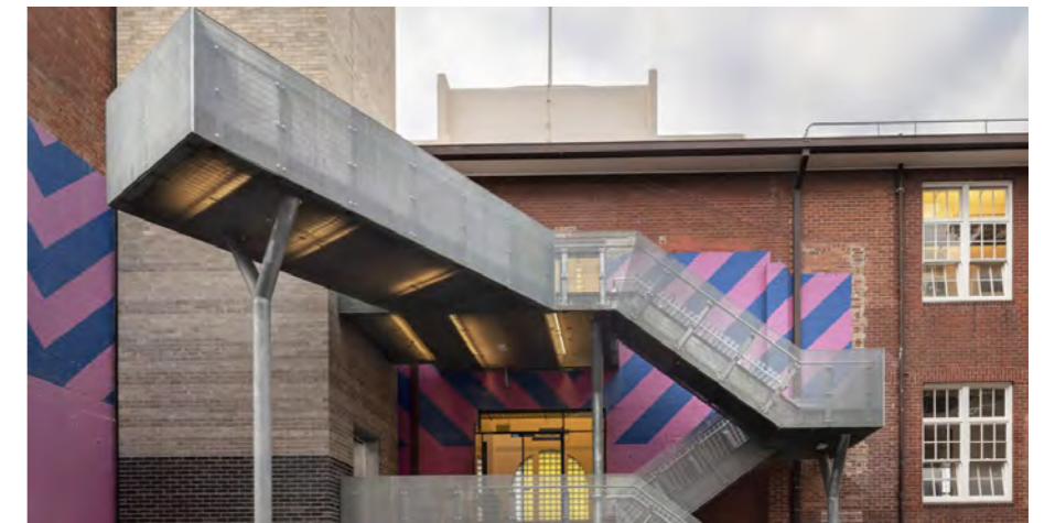
Collingwood Yards, Collingwood - facade works and building additions, with creative uses spilling out into the street and surrounding spaces.
