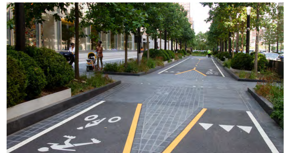
Traffic calming through medians and surface treatments can both increase pedestrian and cyclist connectivity while enhancing streetscape presentations.
