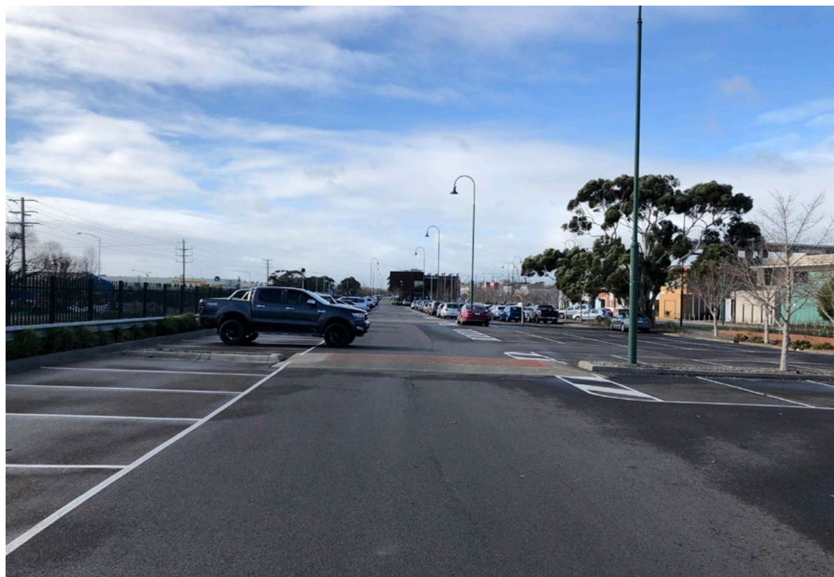
Figure 58: Multi-deck carpark considered over existing at-grade parking west of Council Headquarters building Source: M&PC
