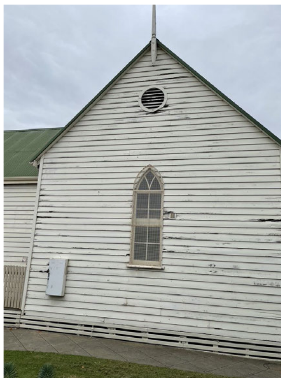
Views of the west side, note typical circular louvred vent in gable end (note visible deterioration to weatherboards at wall corners in the image at right).
