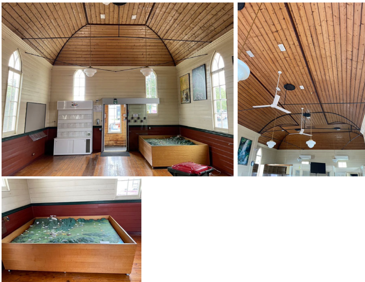
View of the interior looking toward the porch showing covered ceiling and steel rod collar tiles and non-original lights and fans. Note 'Diorama' in corner at right of left image, and bottom left
