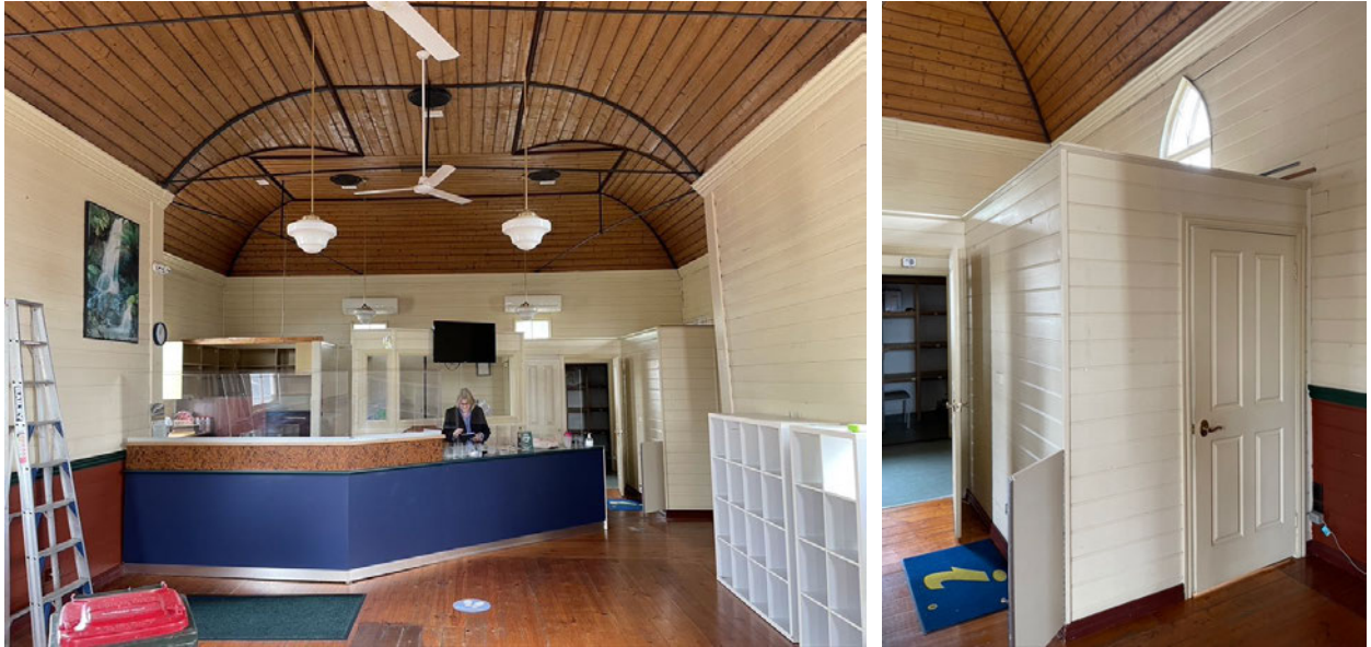
At left, view looking toward the rear showing the non-original counter and partitions installed for the Visitor Centre use. At right, toilet addition.
