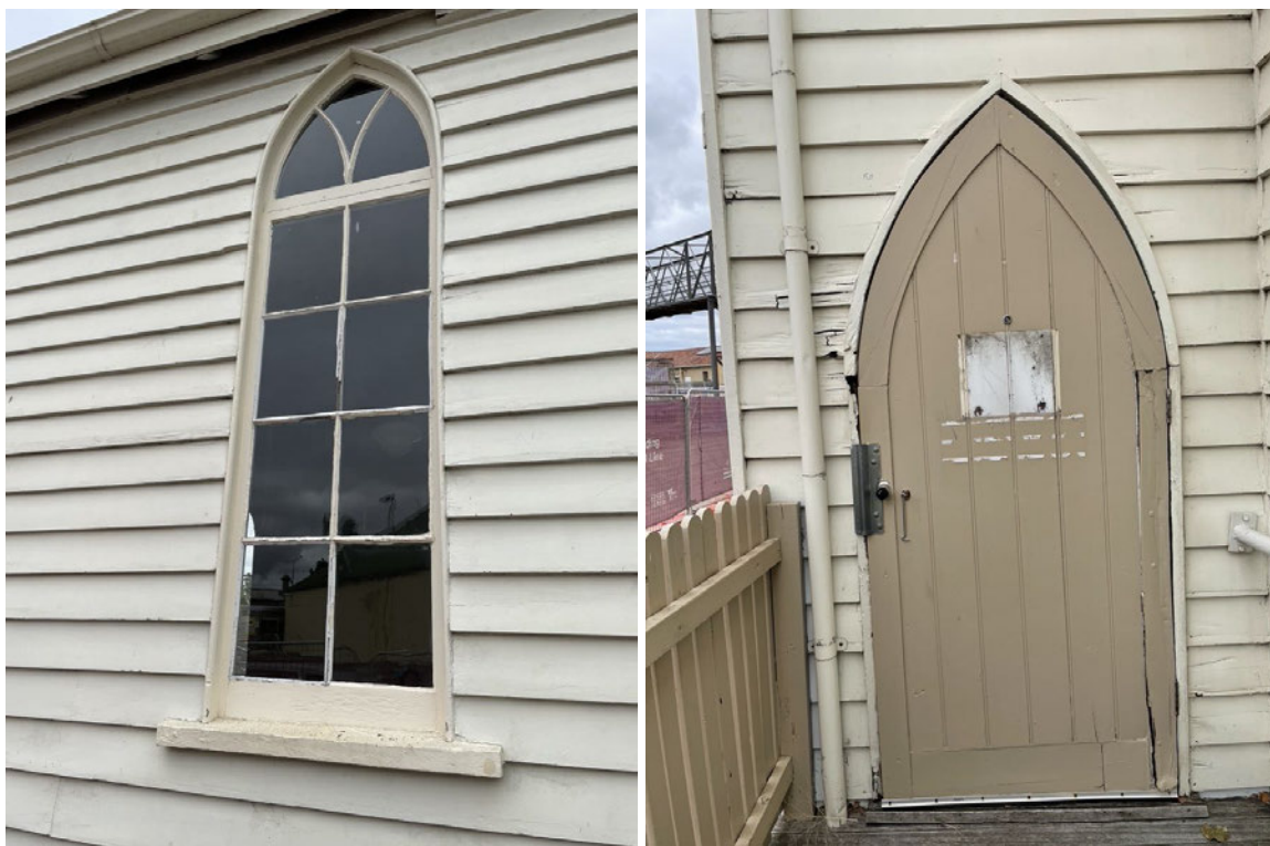
At left, typical window in the 1879 section of the building. At right, one of two doors in the 1888 addition.
