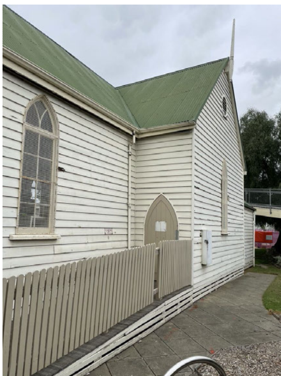
Views of the west side, note typical circular louvred vent in gable end (note visible deterioration to weatherboards at wall corners in the image at right).
