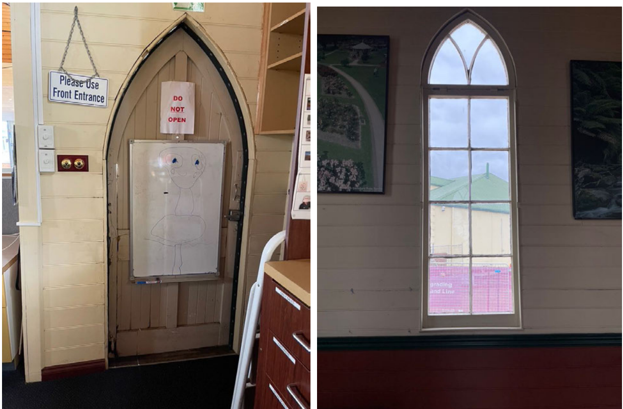
At left, internal view of side door. At right, internal view of nave window
