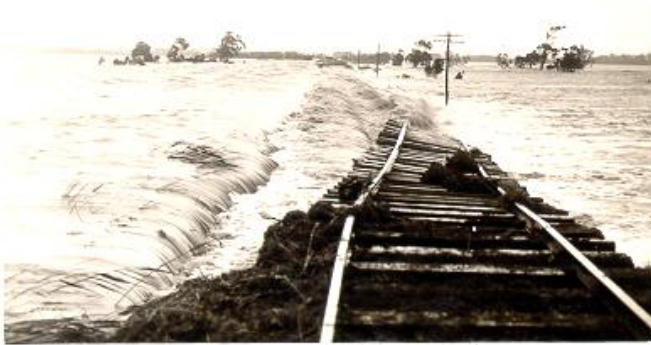
Plate 1 Water overtopping the Traralgon-Maffra railway embankment in 1934 (looking North)
