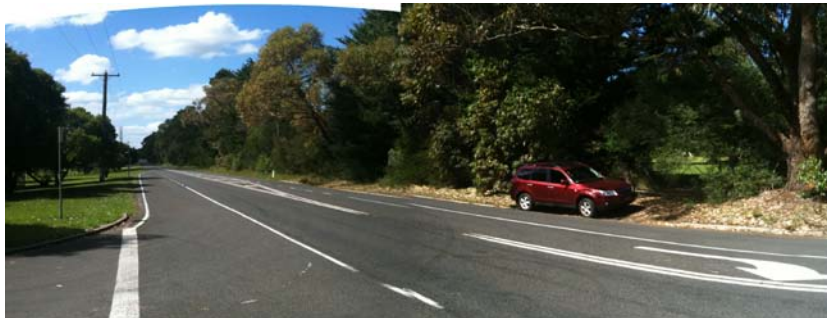
Photograph 7– North-east view down Monash Road (site on right)
