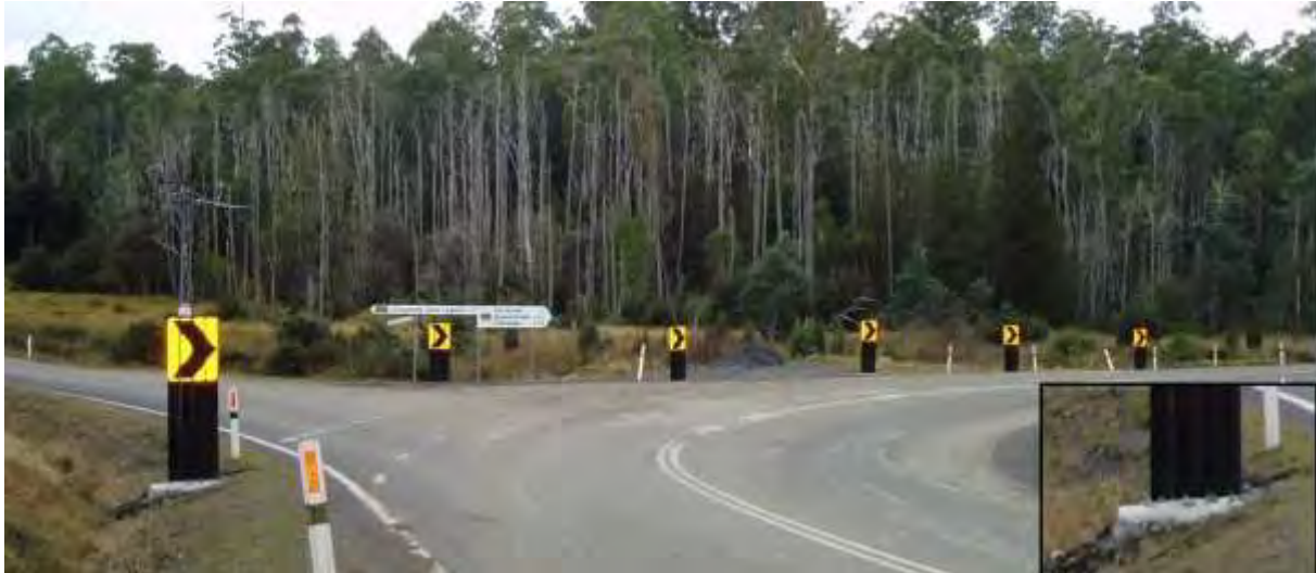
Figure 2 – Collapsible CAM (Tasmania) – inset highlights large concrete base
