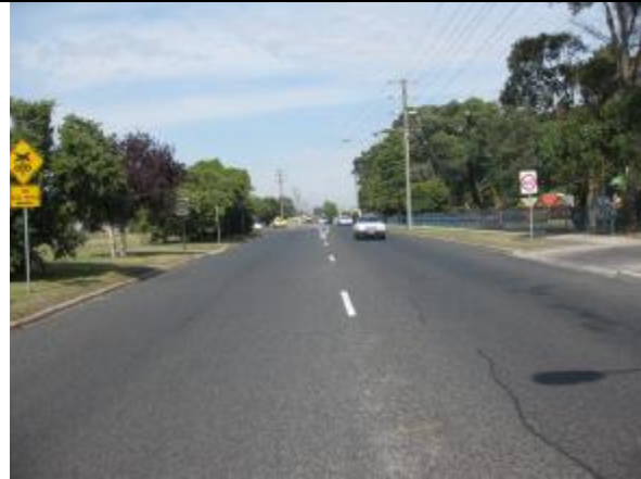
Photograph 3 Waterloo Road east of the intersection with the railway crossing
