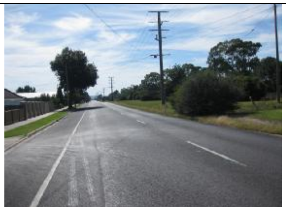
Photograph 2 Waterloo Road west of the intersection with the railway crossing
