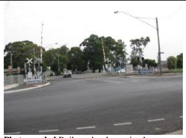
Photograph 4 Railway level crossing between Moe – Glengarry Road and Waterloo Road.
