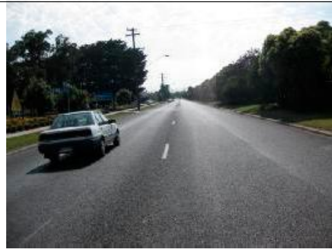
Photograph 6 Waterloo Road east of railway level crossing.
