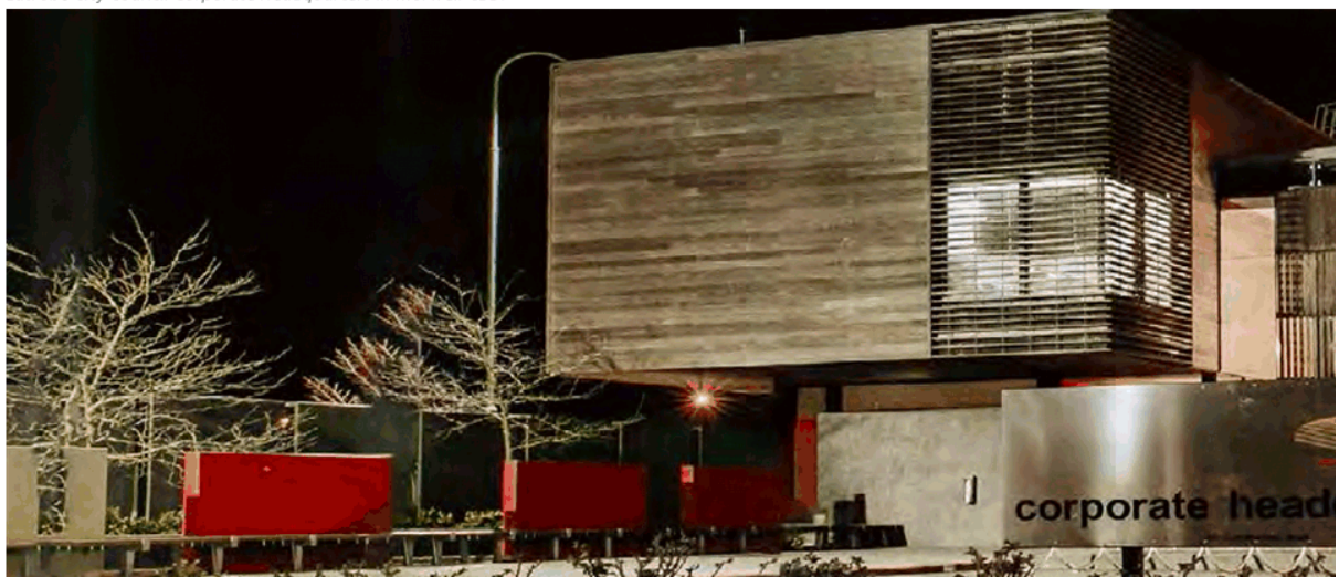
Latrobe City Council Corporate Headquarters in Morwell CBD.
