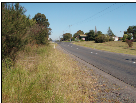
Figure 17: Sight Distance at Proposed Monash Road/Killarney Drive Access - View West
