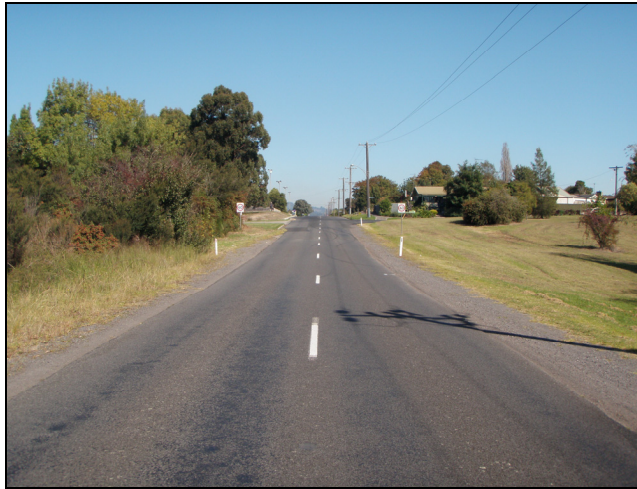
Figure 4: Monash Road Adjacent to Subject Site - View West
