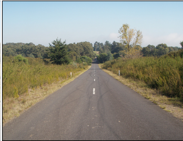
Figure 5: Coach Road Adjacent Subject Site - View West
