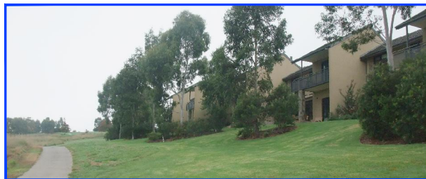
Design guidelines are to be employed at subdivision stage to ensure that dwellings are designed to overlook the shared path network and adjacent golf course
