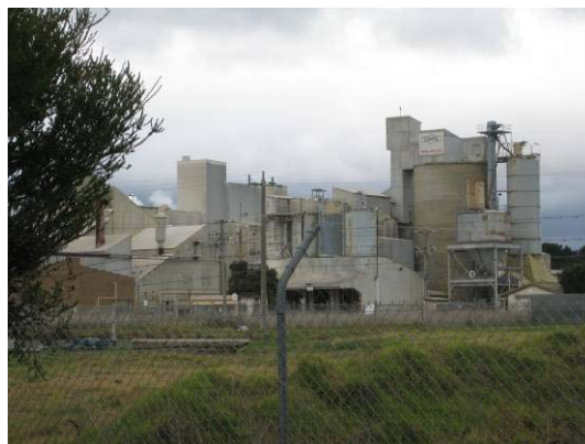
Unimin Traralgon Plant.
