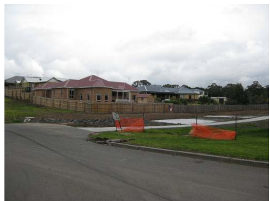
New large format residential development to the south of the study area.
